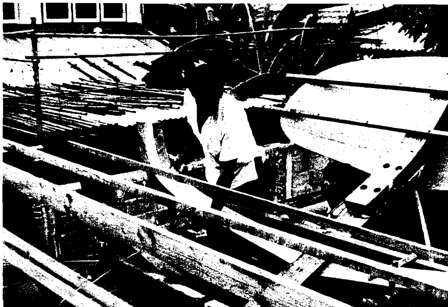
Jeff and Haw framing
