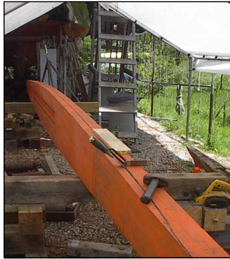
Chisel cuts at stations
